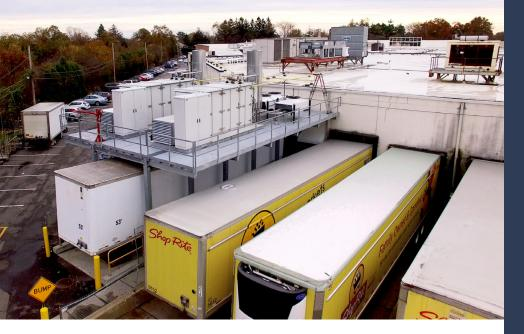
Unison custom-designed a structure to support two CHP engines over an existing high-traffic loading dock.
